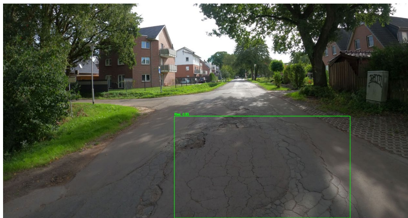
Fig. 2: Exemplary result of the AI model to detect bike path damages
